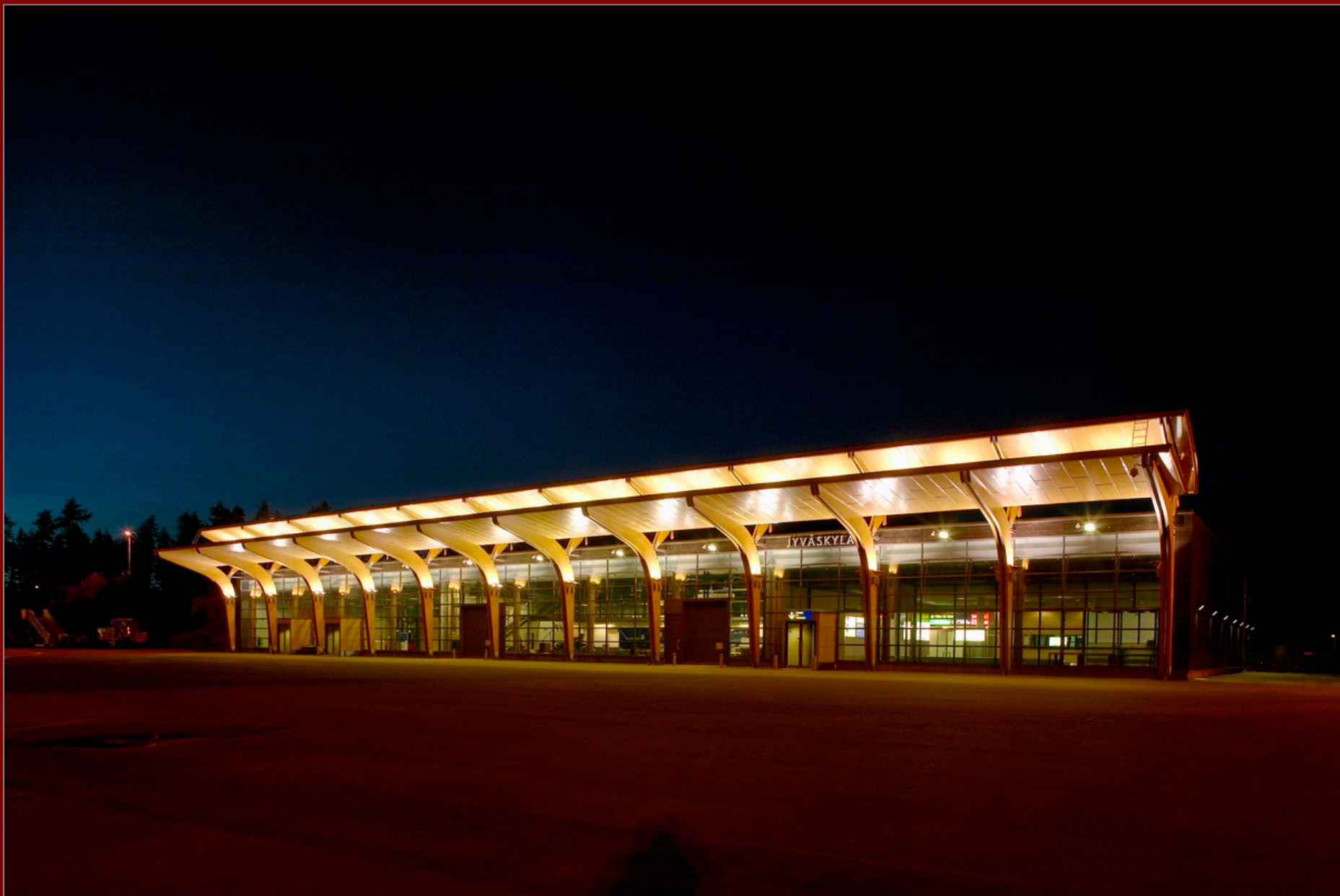
Jyväskylä Airport Terminal
