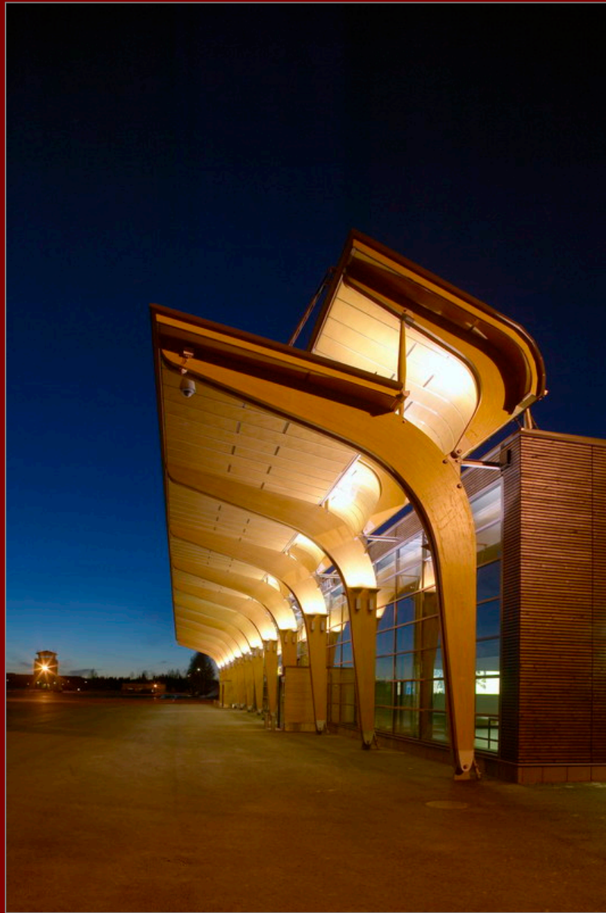
Jyväskylä Airport Terminal
